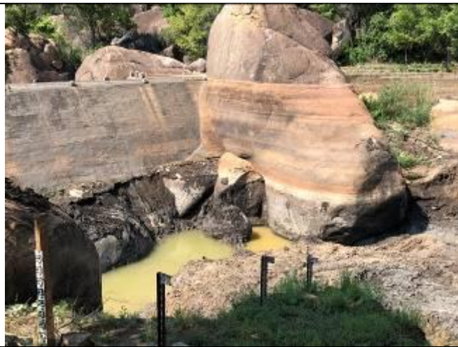
Maleme Dam November 2020
